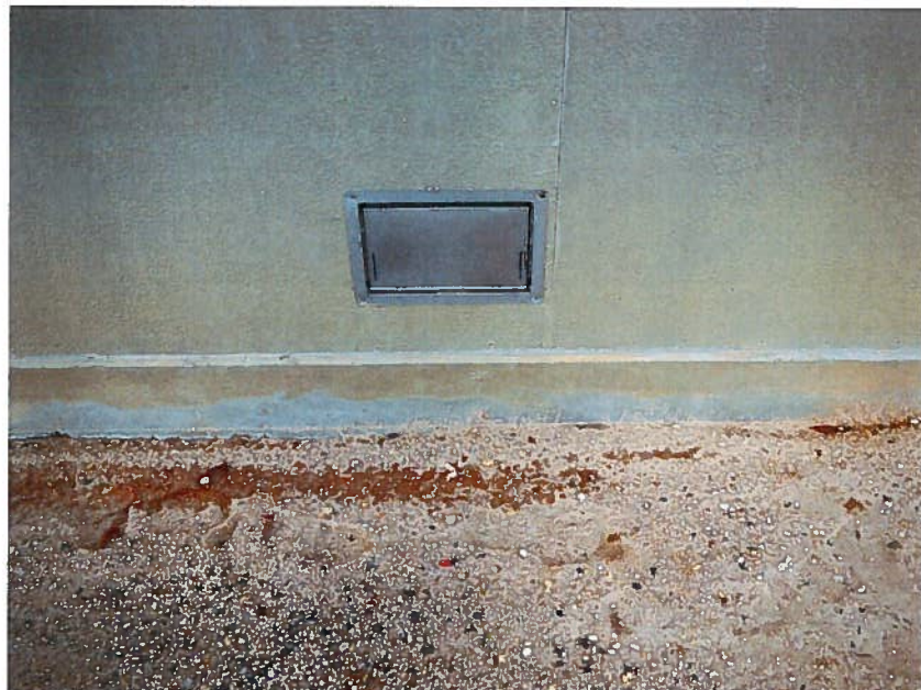
TYPICAL FLOOD VENT 11/14/2015
